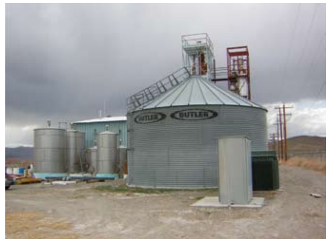
Figure 3. Grain silo, methanol recovery towers, tank farm.
