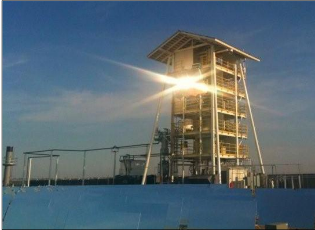
Sundrop Fuels solar gasification-based research and development facility in Broomfield, Colorado.
