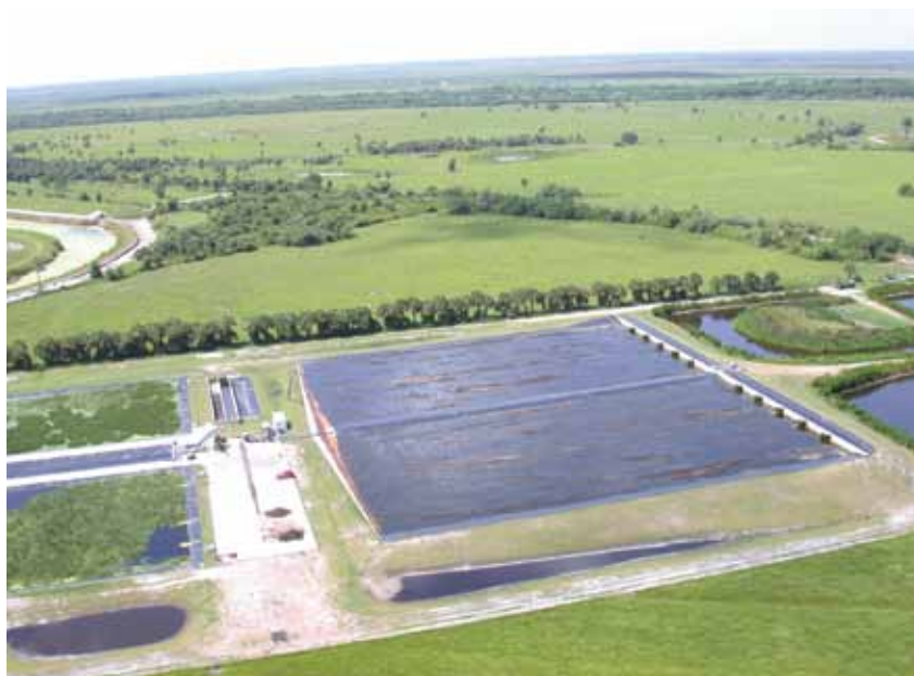
Figure 15: A 2.5-acre algal turf scrubber can provide nutrient control for over 10 million gallons per day.
