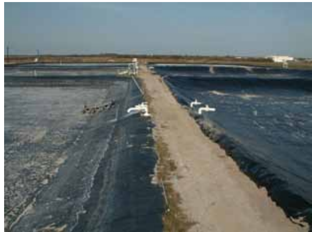
Figure 8: Open ponds often use pond liners to limit water discharge and prevent contamination of culture medium.
